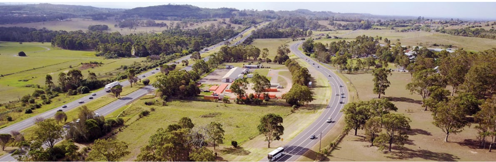
Existing traffic on the Hume Motorway and Menangle Road
